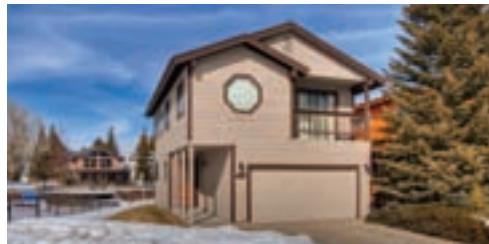
Slalom Court – Classy custom remodel from top to bottom is offered from this 4 bedroom, 3 bath downstairs living layout with 2085 square feet of living. $749,000
